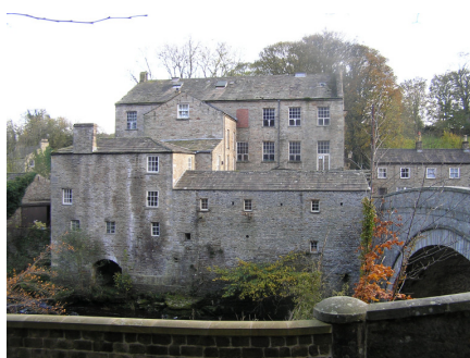
Yore Mill, Aysgarth Falls: small scale hydro electricity generation project. (©YDNPA)
