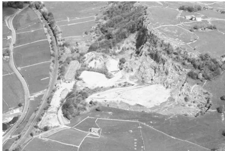
Hoffmann Kiln and a disused limestone quarry, Langcliffe. (YDNPA)
