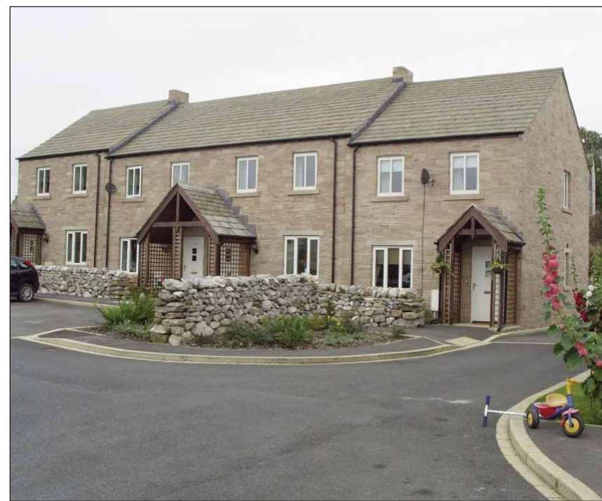
New buildings designed to reflect traditional styles, Garrs End Lane, Grassington (YDNPA)
