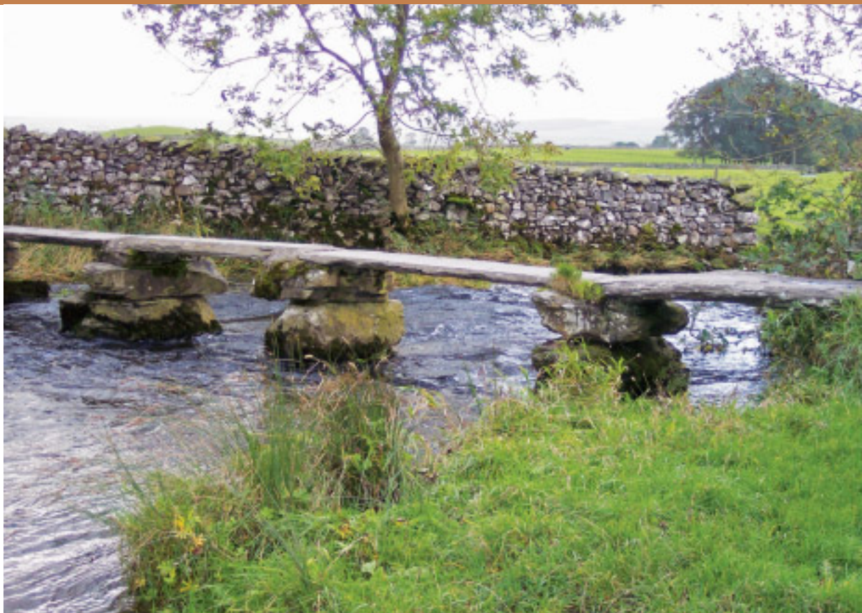
Flascoe Clapper Bridge, Austwick – these simple forms of crossing consisted of piles of stones with slabs across the top.
