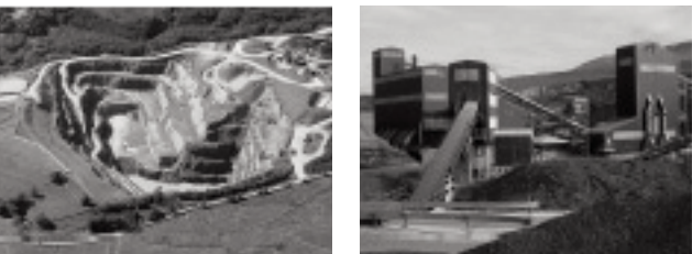
Ingleton Quarry. Aerial view. (Hanson Aggregates).
