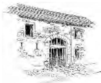
By exploiting the openings of a barn its functional character is retained
