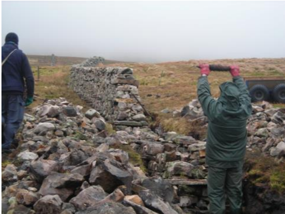
Photograph 8 - wall restoration ©YDNPA
