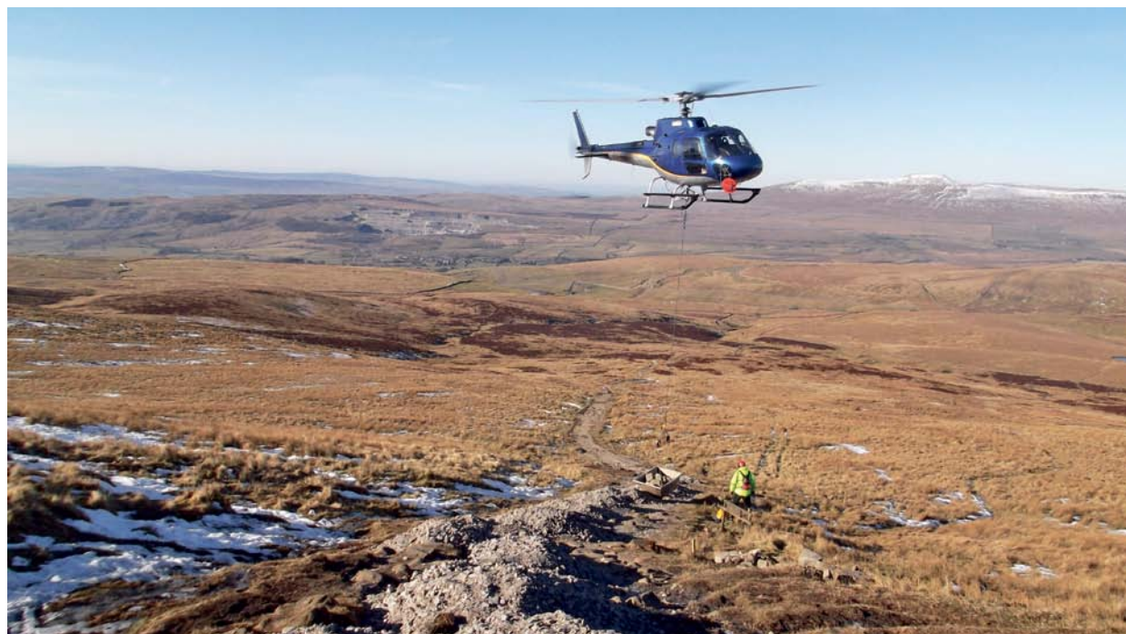
Above: Limestone pavement on the Pennine Way above Malham Cove. Below: Airlifting stone flags for footpath repairs
