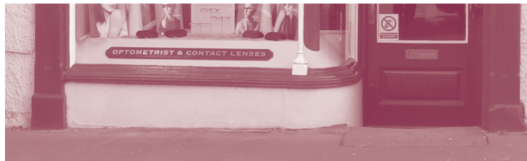
Typical rendered stallriser, protected by intricately moulded sill above, as found throughout South Lakeland
