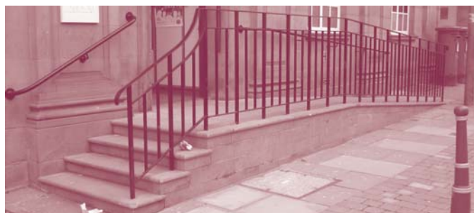
Sometimes ramps can be considered to ease access for those with mobility devices such as wheelchairs. The ramp has a shallow gradient and the handrail provides extra support and safety
